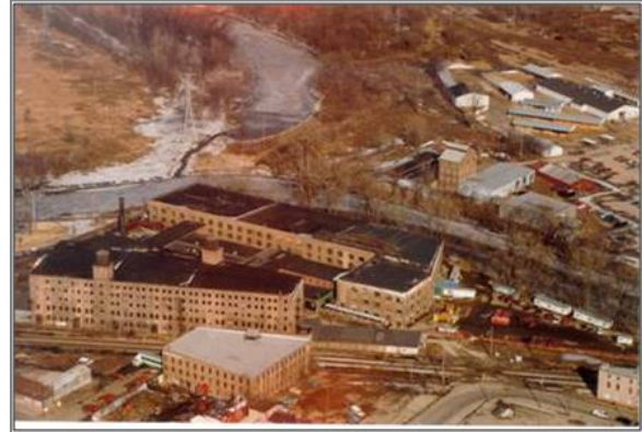
Before: Burgess Battery Brownfield Site
